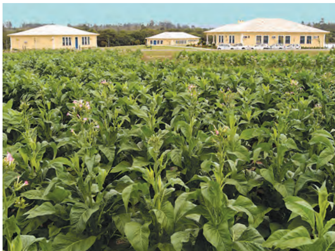
The view from the north side of ULT's main Training, Administrative and Laboratories building at the Experimental Station.
